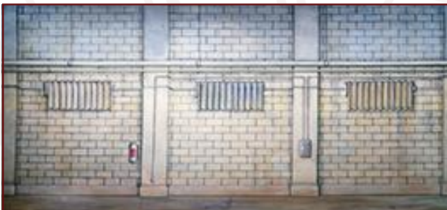
30-IA. Basement 43' x 21' - 37 lbs Typical basement with radiators.
